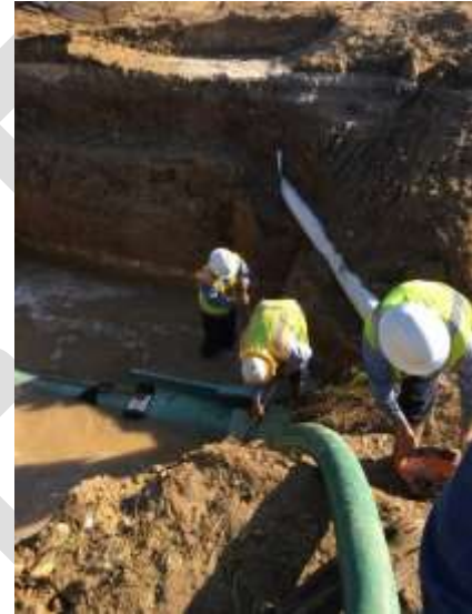
Roma Public Utilities Dept. repairing water line.
